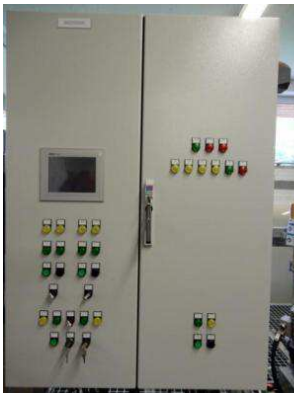
Fig. 2: Control cabinet with operating display
